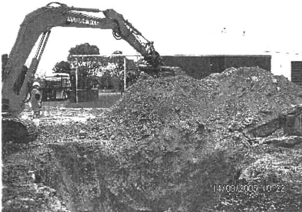
View to the North of the site.
