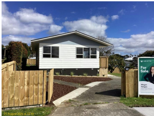
Front access / driveway
